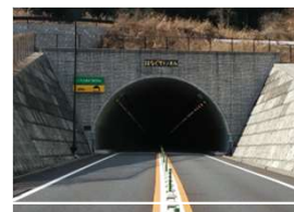
Number of Road Tunnels 562 (as of Mar 31, 2021)
